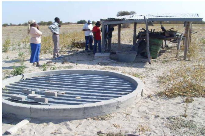
**Plate 3: Existing water harvesting structure and underground water storage tank (Mopipi)**
